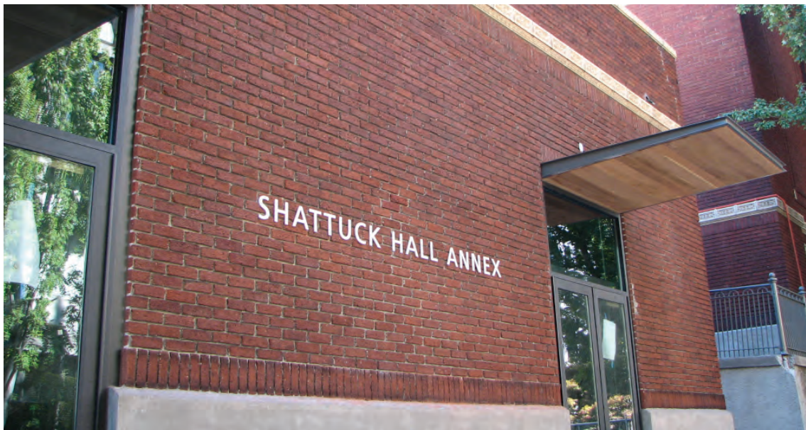
Renovations of the Shattuck Hall Annex
