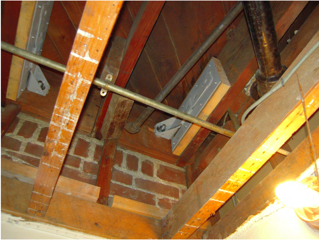
Figure 6.3 Example of a floor joint tie back in Trinity Place Apartments
