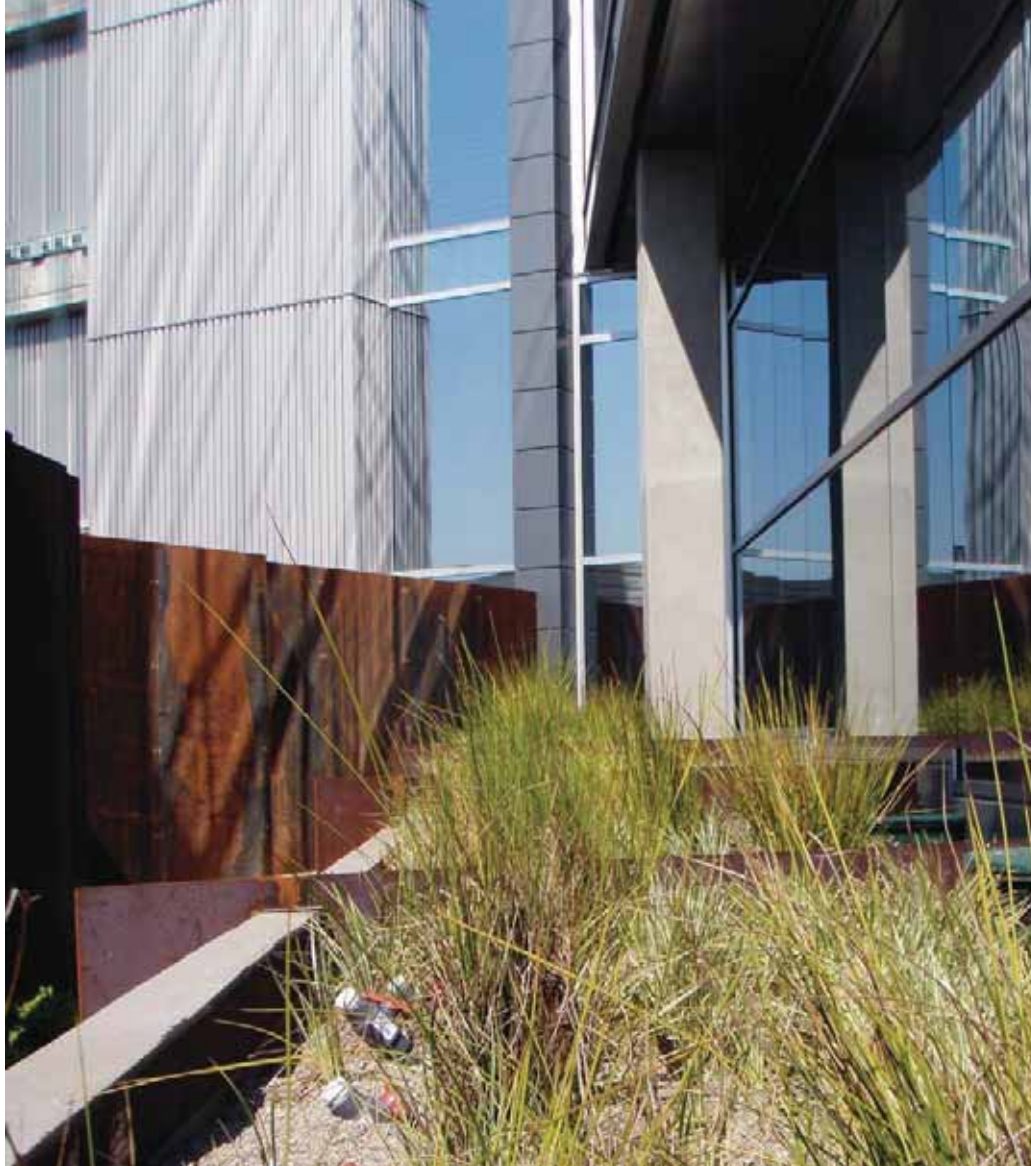
Outdoor treatment tanks of the Port of Portland's Living Machine.
