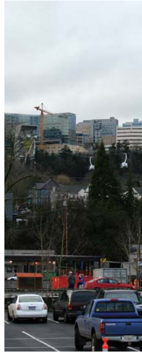
The new tram connects OHSU's upper and lower campuses.
